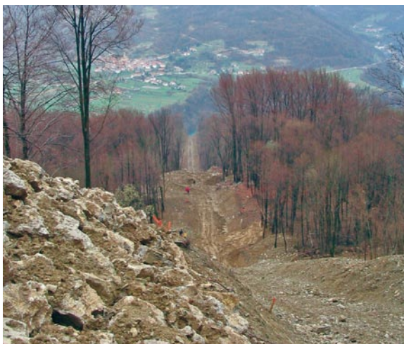
View along the alignment of the penstock
