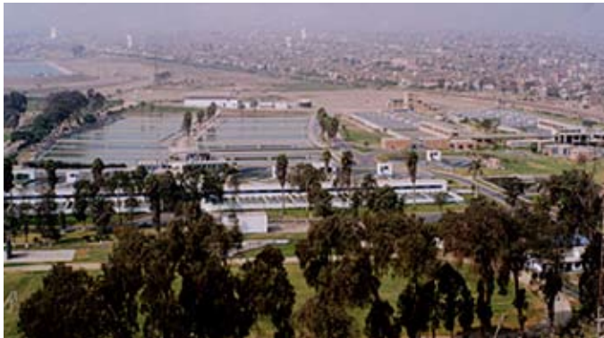
Abwasserreinigungsanlage am Rimac-Fluss, Lima Rimac River Waste Water Treatment Plant, Lima
