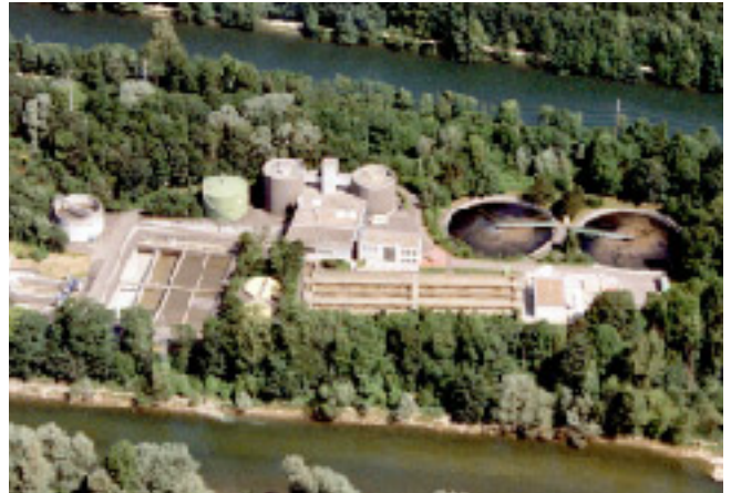
Abwasserreinigungsanlage ARA Olten in Winznau/Schweiz Sewage treatment plant STP Olten in Winznau/Switzerland
