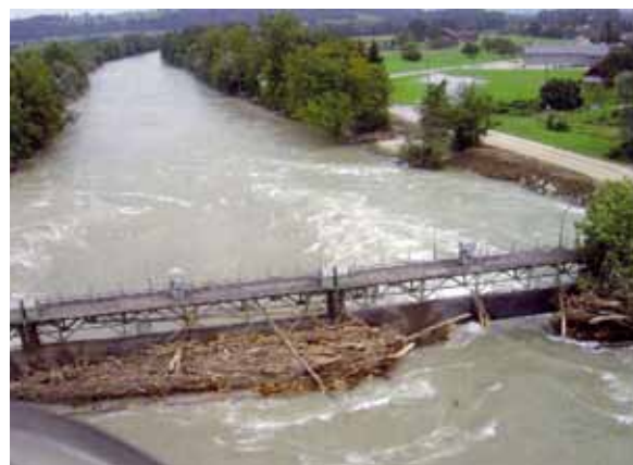
Driftwood pile in Emmen (left) and log jam at the Perlen weir (right) during the flood of 2005
