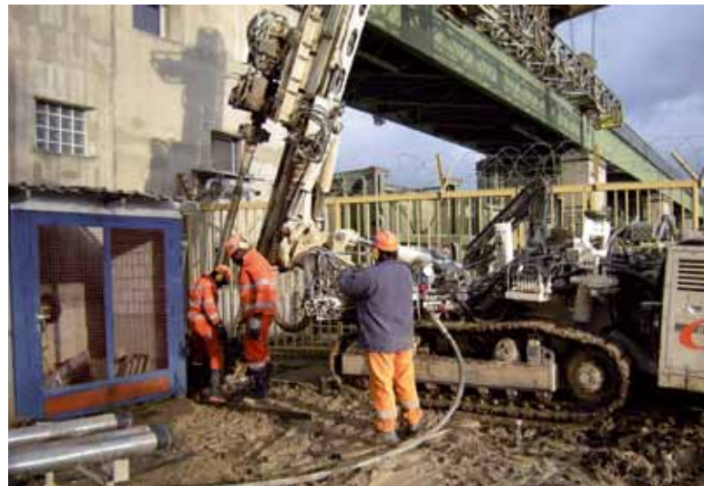
Drilling operations (right), Drilling machine, Tube-à-manchette (left)
